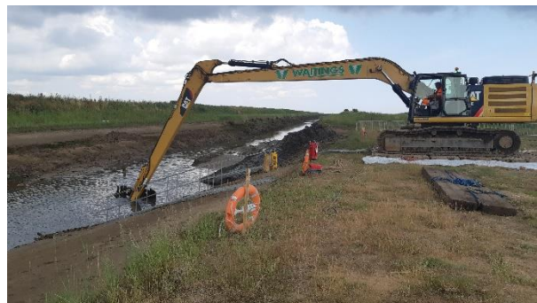
Piles being removed
