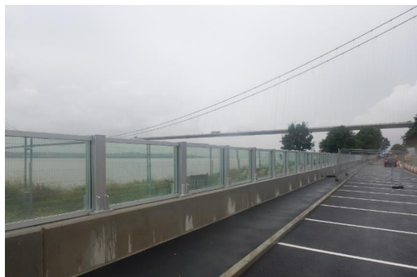
Stage 3 Wall progress showing installed glass panels
