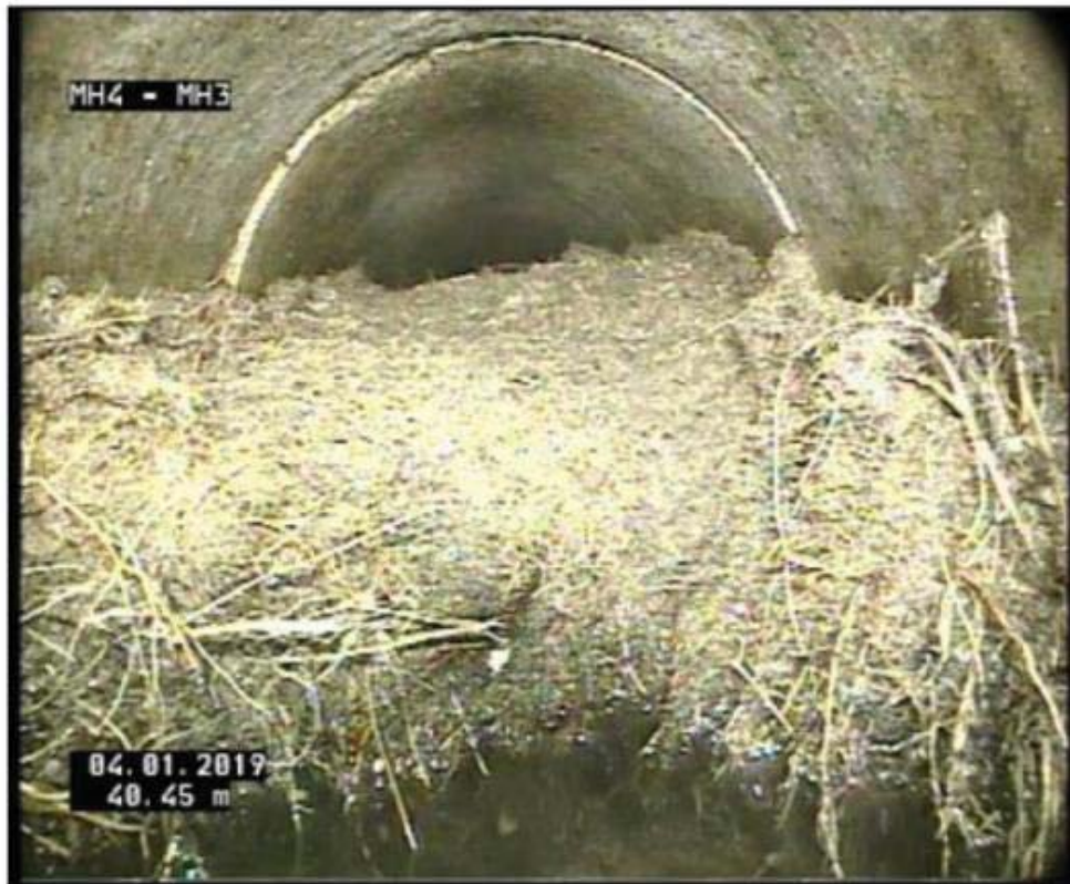
Photo: 2_1_12_10012019_144159_A.jpg 39m, Roots, mass, 80% cross-sectional area loss
