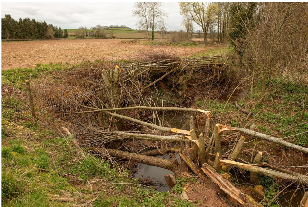
Photo 9: Hedge laying and revetment work on the River Lodon opening up a shaded part of the river
