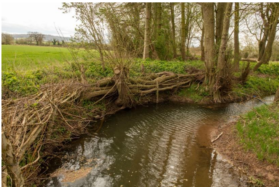
Photo 5: River revetment work to stabilise the bank and provide wildlife niches
