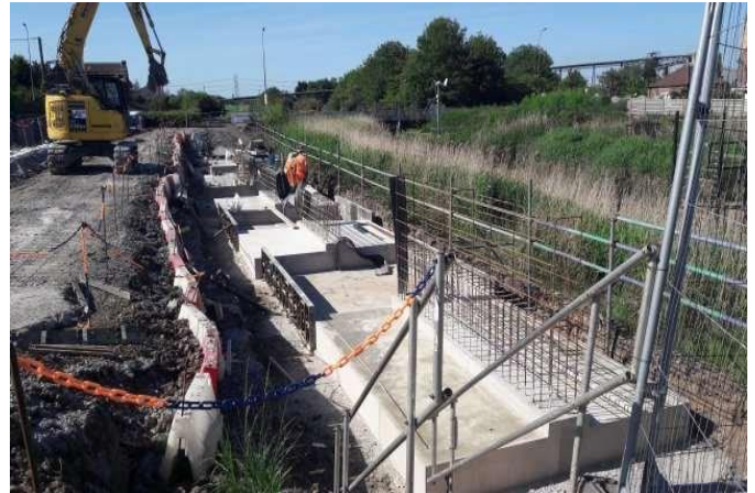
Flood wall foundations being cast along East Drain
