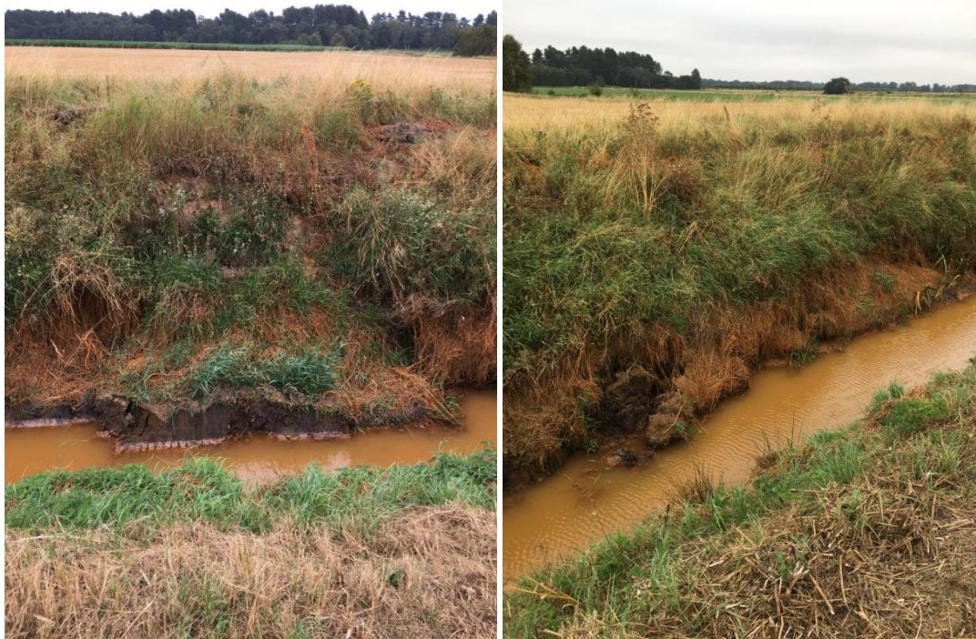
Two slips on Jenny Hurn Drain, not impeding flow
