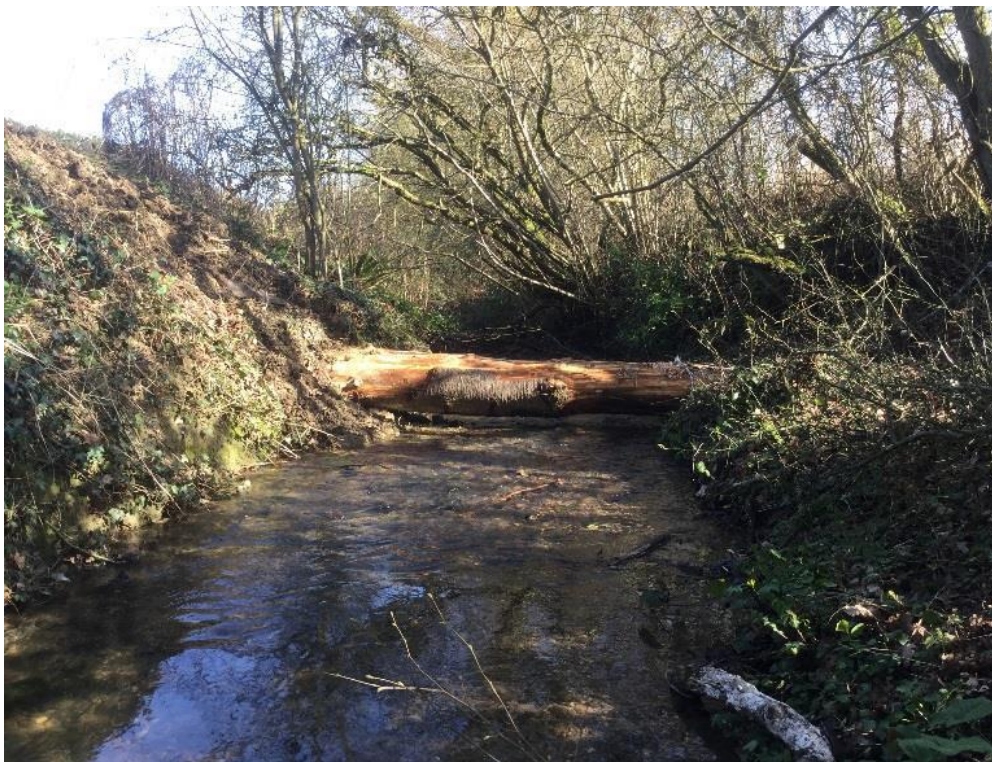
Woody dam in Littlestock Brook
