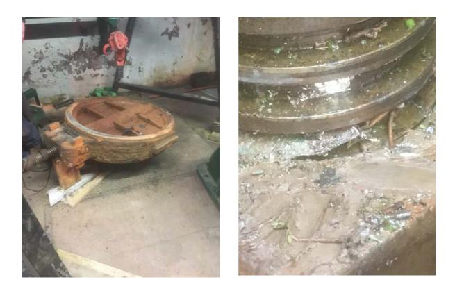
Perry's pumps have removed the bronze shaft and nut and are being machined before replacement. Costs and timescales are being determined with the Contractor.
