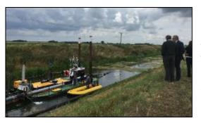
• South Forty Foot Drain Cutter Section de-silting works: Black Sluice IDB, on behalf of the EA, have completed the first phase of works to increase flow and capacity in the SFF Drain through a de-silting regime. We are currently finalising Phase 2 of these works.
