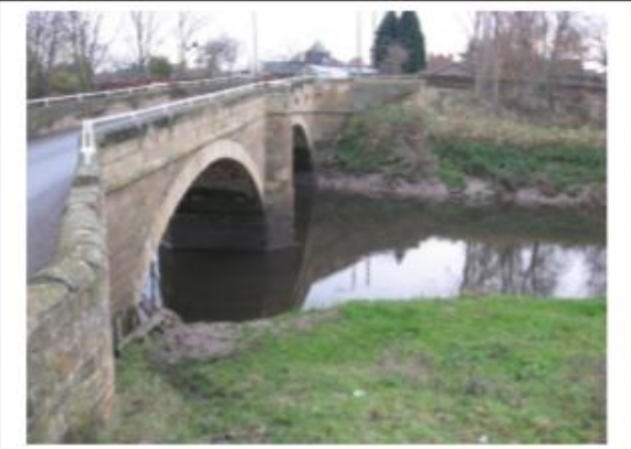
Stainforth Bridge Normal Flow
