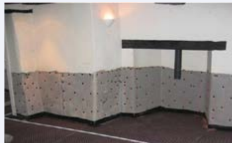
Figure 3 Internal walls now covered with a mesh membrane, and floors are covered with a studded membrane
