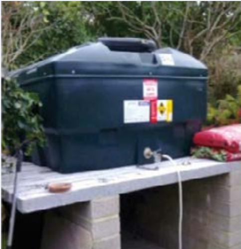
Figure 3 Fuel oil tank on raised plinth
