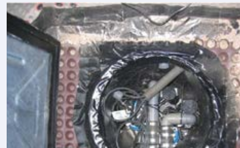
Figure 4 Two sumps (similar in size to a domestic dustbin) contain pumps designed to operate at different water depths.
