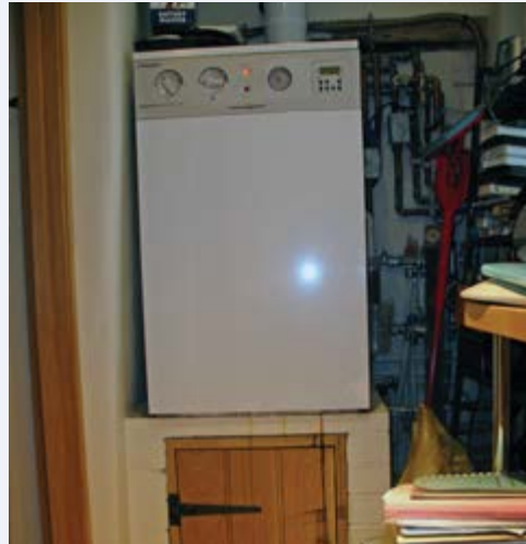
Figure 4 Boiler on plinth
