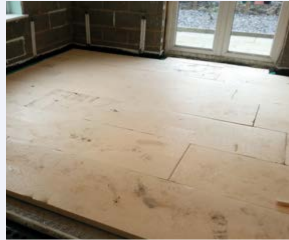
Figure 6 Closed cell (waterproof) insulation on the floor
