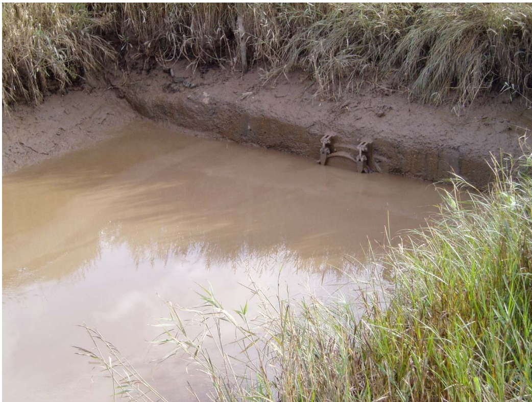
Picture 2: 29 September 2017 siltation covering outfall
