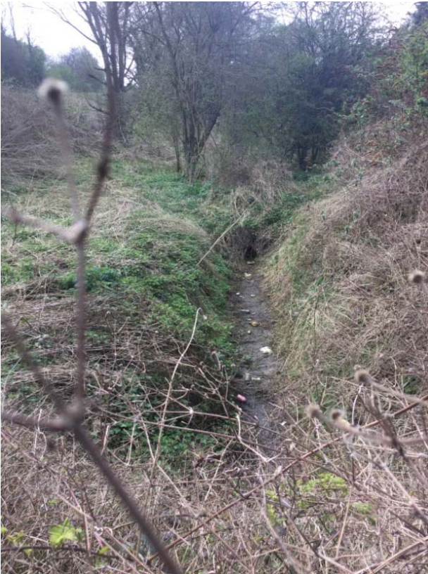
4. Upstream of Waterside Drain as viewed from Quay
