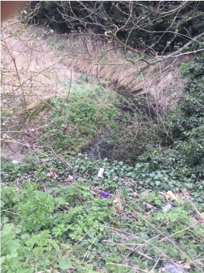
1. Downstream of culvert under
