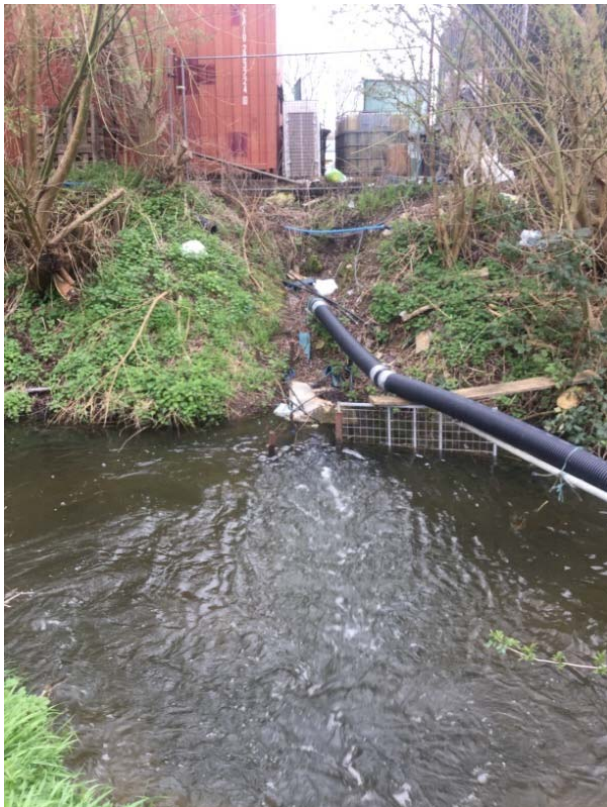
The water velocity is driven by an 18" diameter plastic ridged pipe discharging water from Marina dry docks to the extent it has eroded the opposite bank. The Board consented this discharge several years ago.
