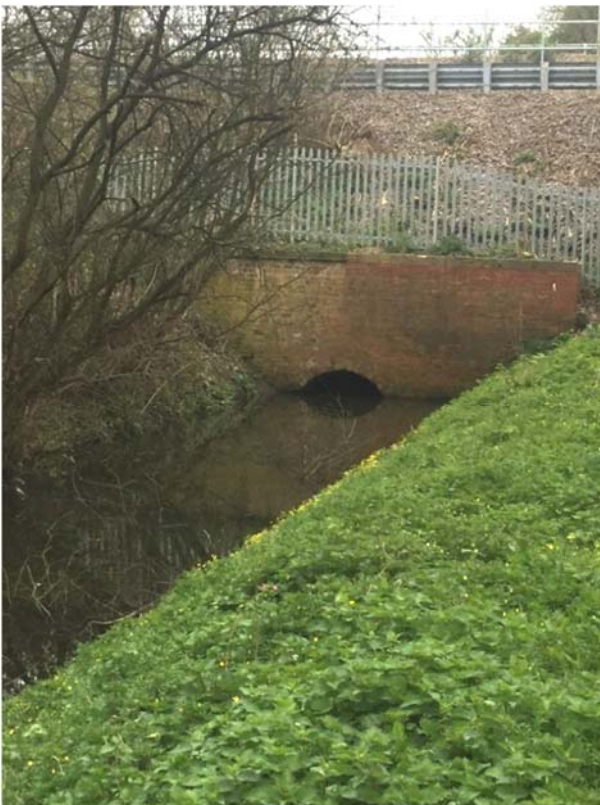
Culvert under railway.
