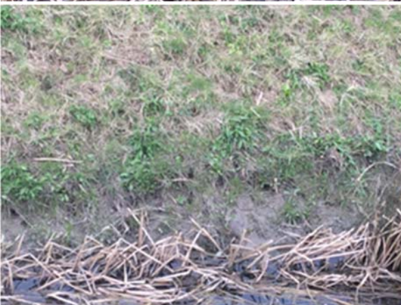
Whilst several burrows were noted, no evidence of latrine was seen however the burrowing is extensive to the rear of the piling boards, latrines may occur there as there is no obvious area available in front of the toe piling. One recently killed water vole ( Arvicola amphibious ) was noted, the method of execution, bitten at the back of the neck, suggesting a weasel or stoat
