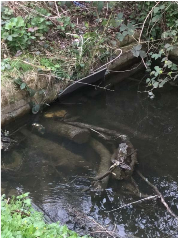
Branches upstream of footbridge
