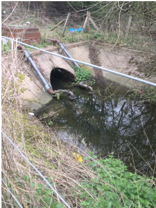
Storm pipes in bed of drain from Omega Boulevard.
