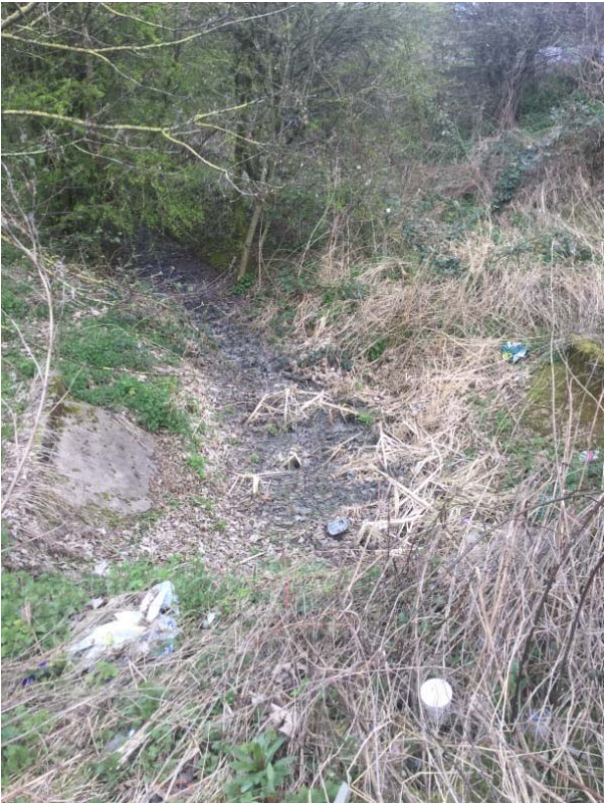
2. Upstream side of watercourse dry.
