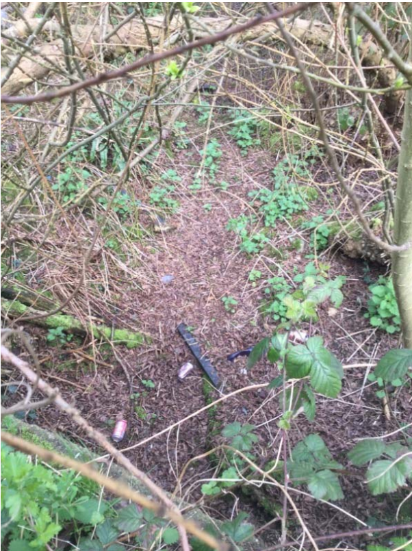
5. Downstream Waterside Drain as viewed from Quay
