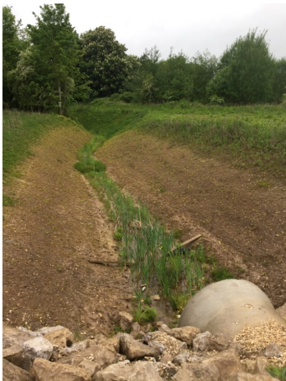
Drain upstream of track over Anderson Road Drain
