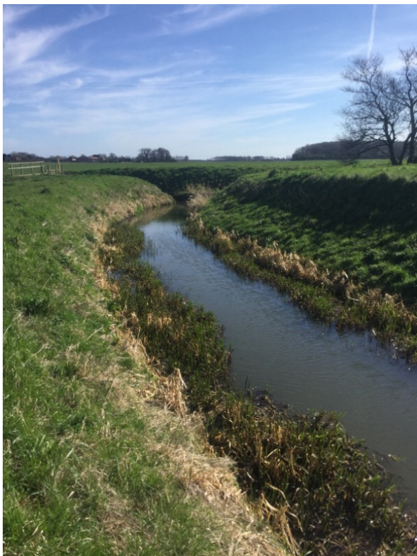
Township Drain before junction with Downes
