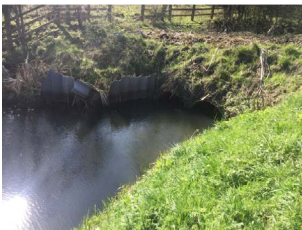
adjacent M62 culvert
