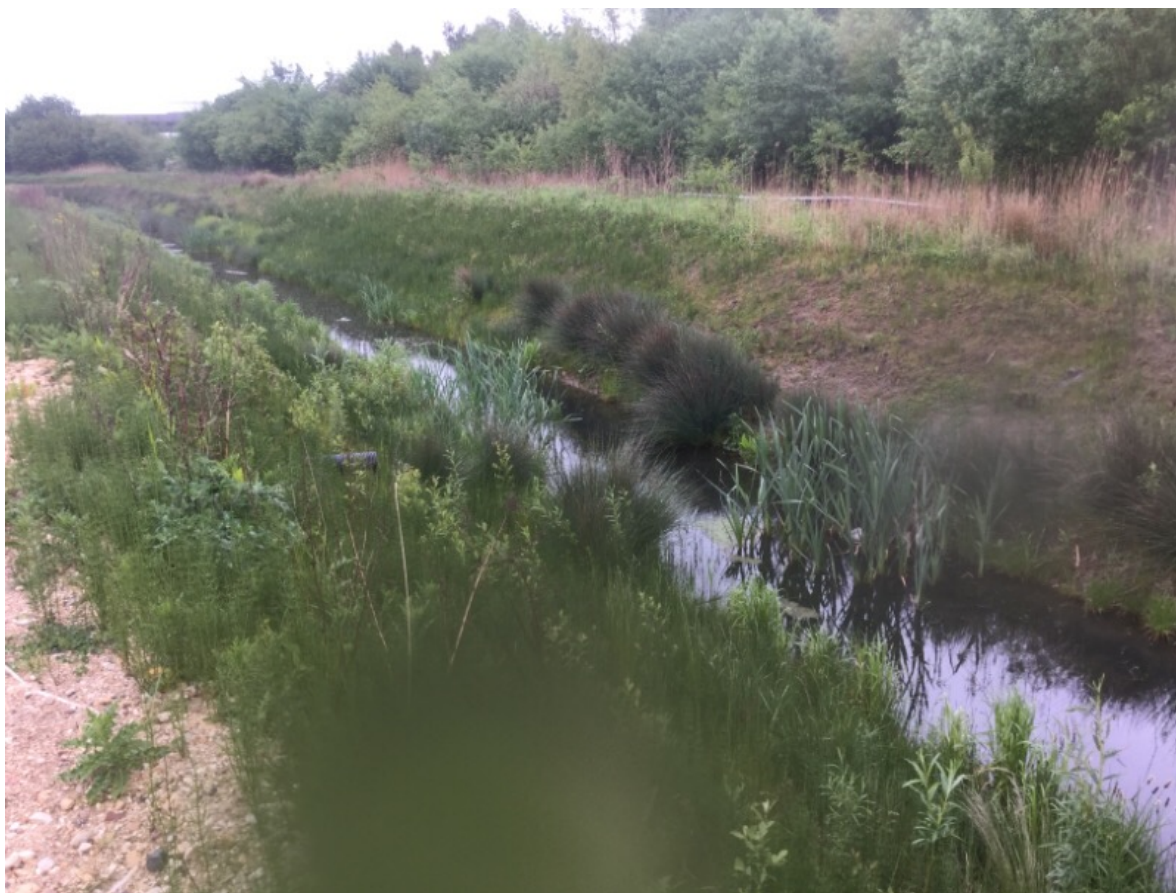
Bank side vegetation growing well in places
