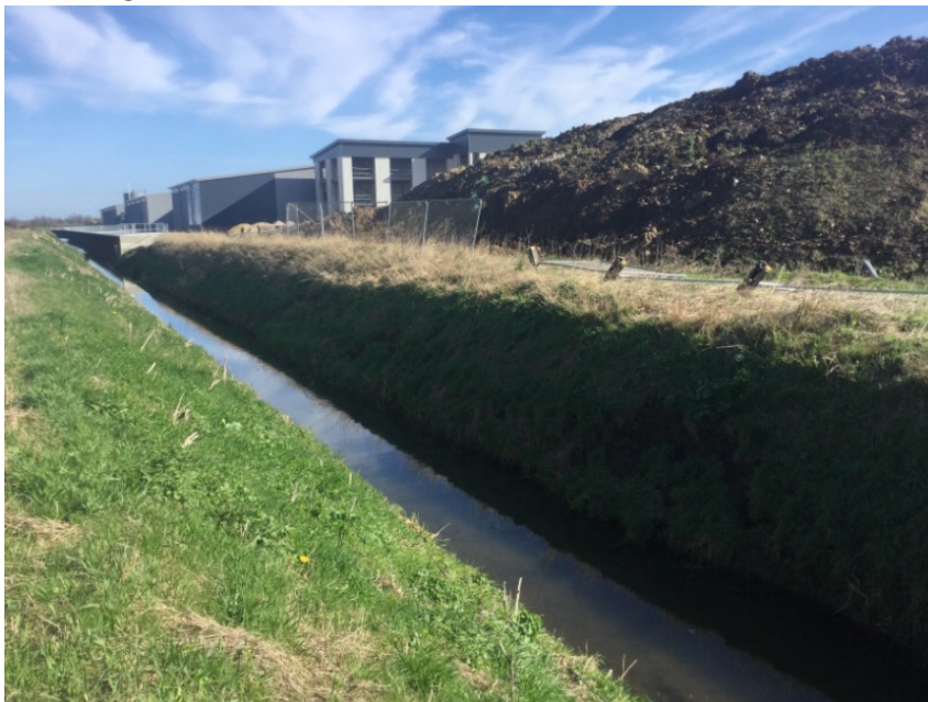
Township Drain adjacent
