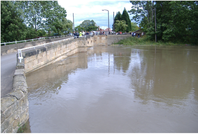
Stainforth Bridge Flooding Event
