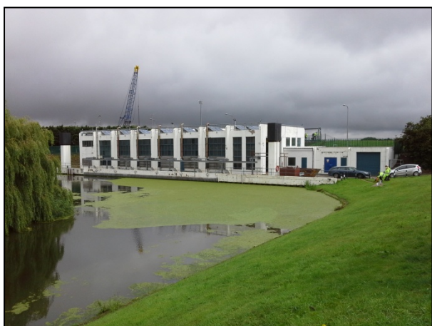
Keadby pumping station
