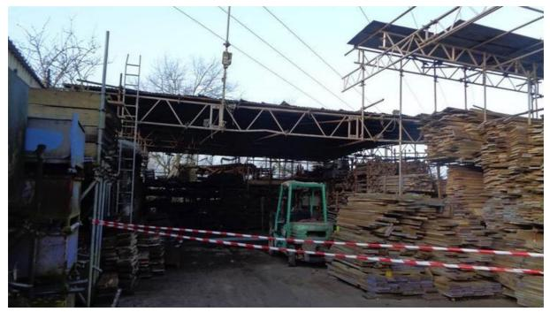
The scaffolding erected close to the overhead power lines. Image: HSE Swindon Magistrates' Court was told that the structure touched 33 kV overhead power lines on 19 December 2016.
