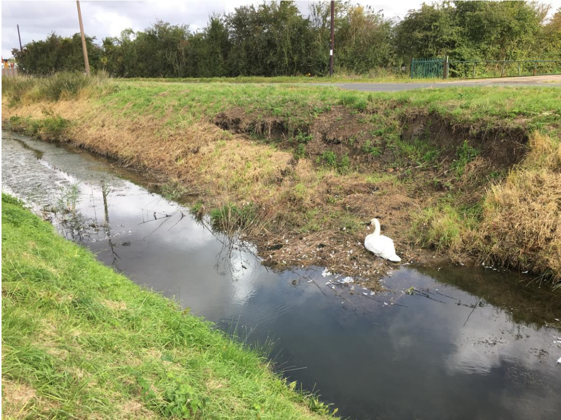
Figure 2: slip facing north east
